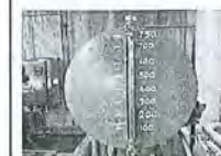
Item No. 2.5 Check diesel level of Engine
