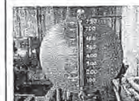
Item No. 2.5 Check diesel level of Engine
